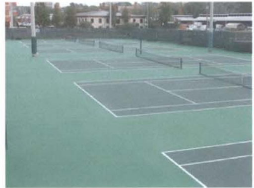
The Florida State University Tallahassee, FL Scott Speicher Tennis Center 12 asphalt courts
